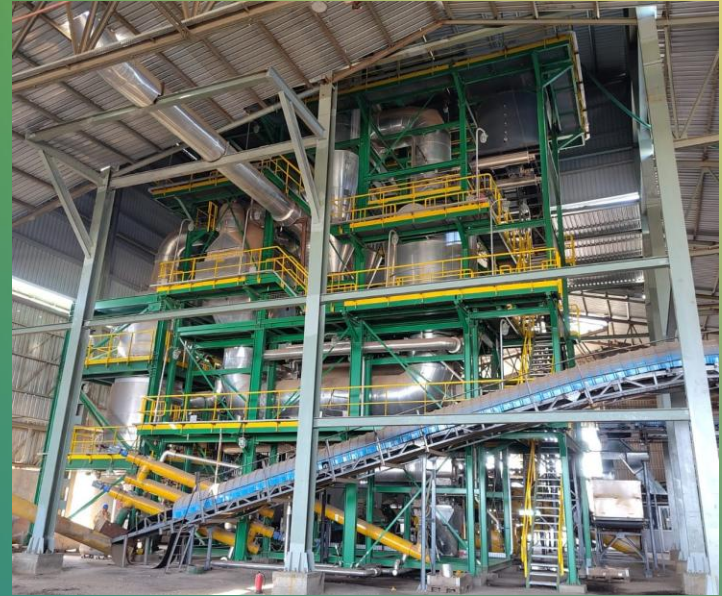
Commercial plant. Capacity: 4.0 ton per hour
